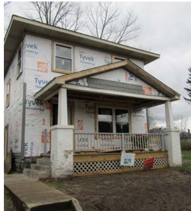
Rehab Construction Homeownership: 750 Harrison Ave
